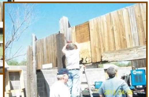
Mike Horton on the ladder pounding the 2x8 piece beside the steel column, with Mike Bromhall and Ed Dotson watching.
