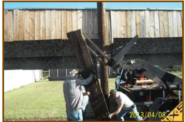
Jim Wilson, Ed Dotson and Mike Horton locating the 2nd tie pair in front of a overhead baffle column. Mike Bromhall is running the skid-steer to hold the ties up.
