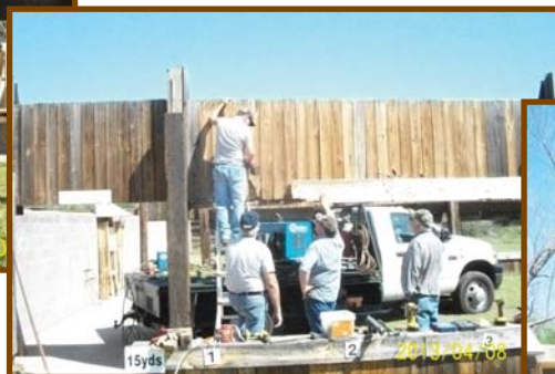
Mike Horton on the ladder, screwing some 2 x 6's in place on the overhead baffle that had been shot up, being watched by Mike Bromhall, Ed Dotson and Jim Wilson.
