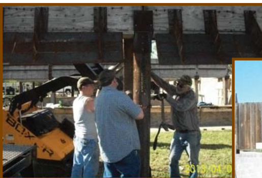
Mike Horton, Ed Dotson and Jim Wilson securing the tie pair in place.
