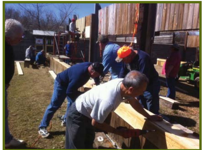
New boards for the baffles
