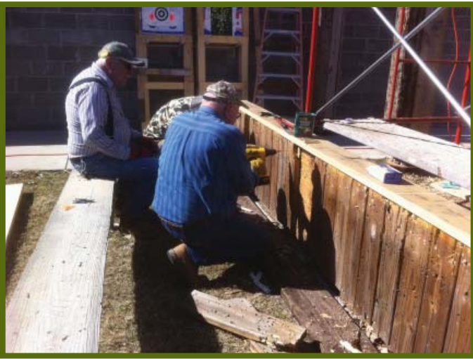
Jim, Kerry and Terry replacing short boards
