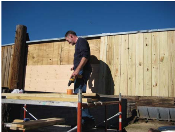
Jeff Zwiebel refacing the upper baffle
