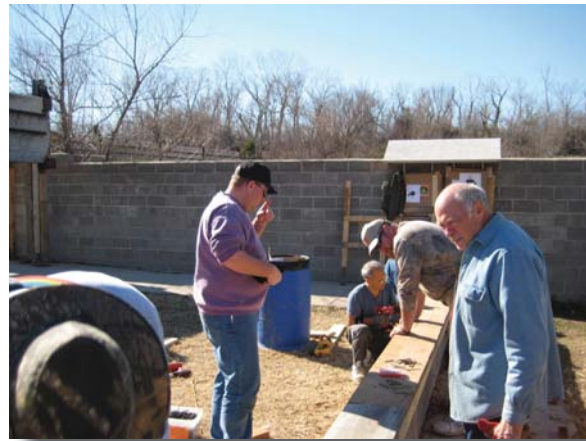
Kirk, Hoa, Dale & Dan re-building the ground baffles
