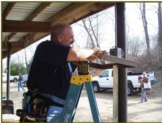
Electrician working on pistol range
