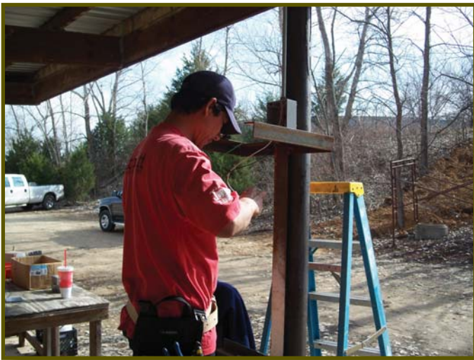
Electrician working on pistol range
