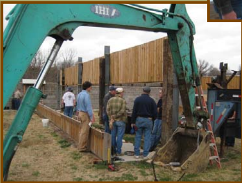
Unloading RR ties with Don Yeandle's excavator, 02 05 09
