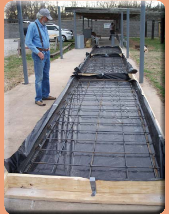
John Slocum looking at forms for rifle range ground baffles.
