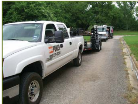
Replacing power line to well
