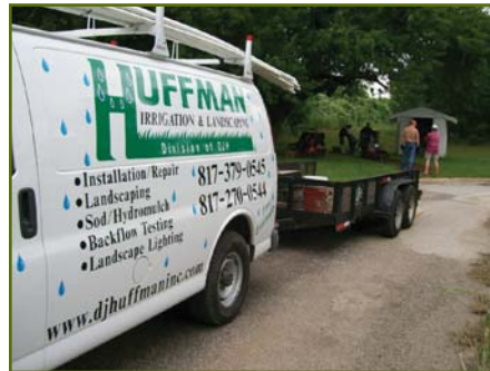
Jason Huffman trenching power line
